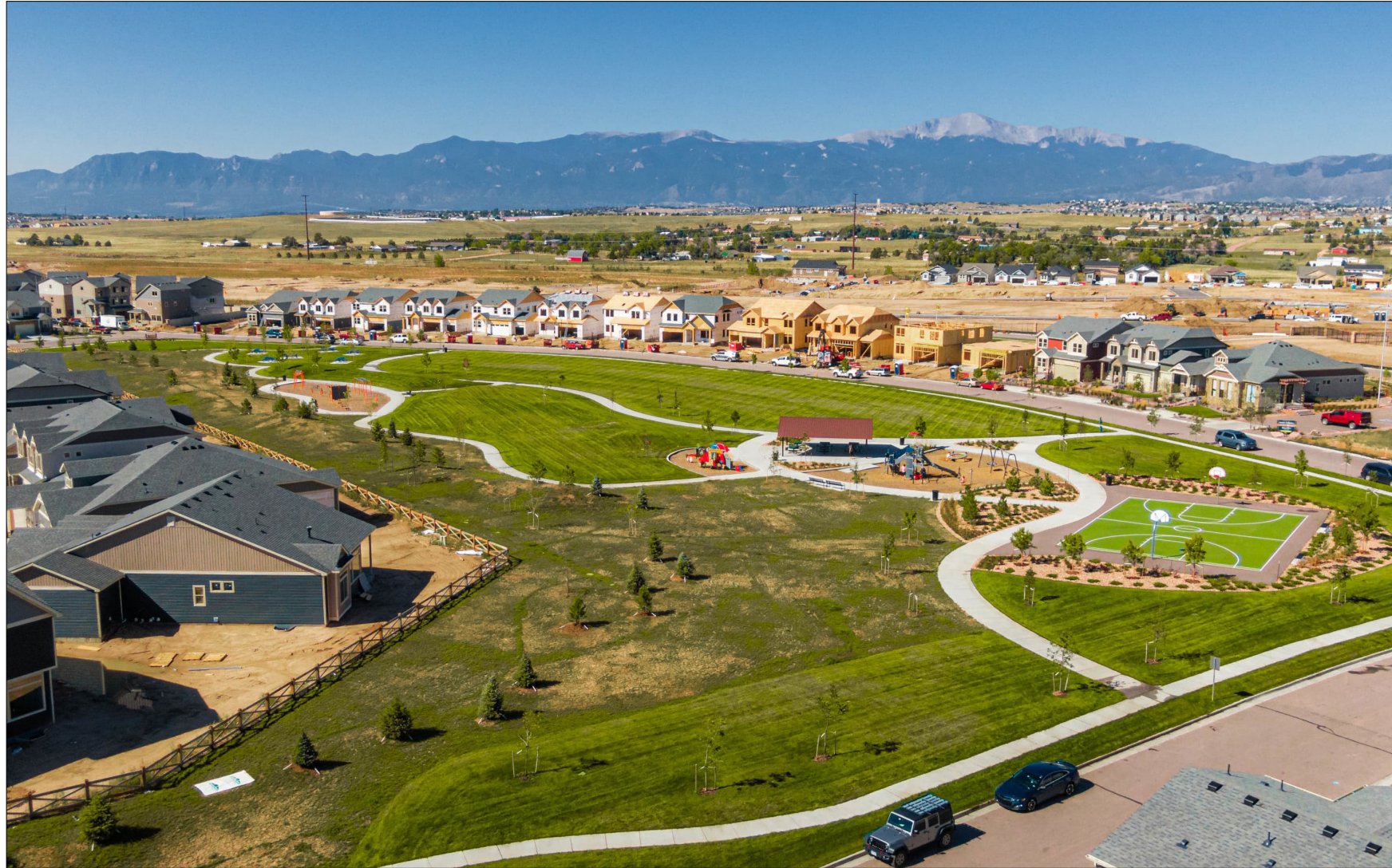
Banning Lewis Ranch Village 3's newly constructed neighborhood park looking west
