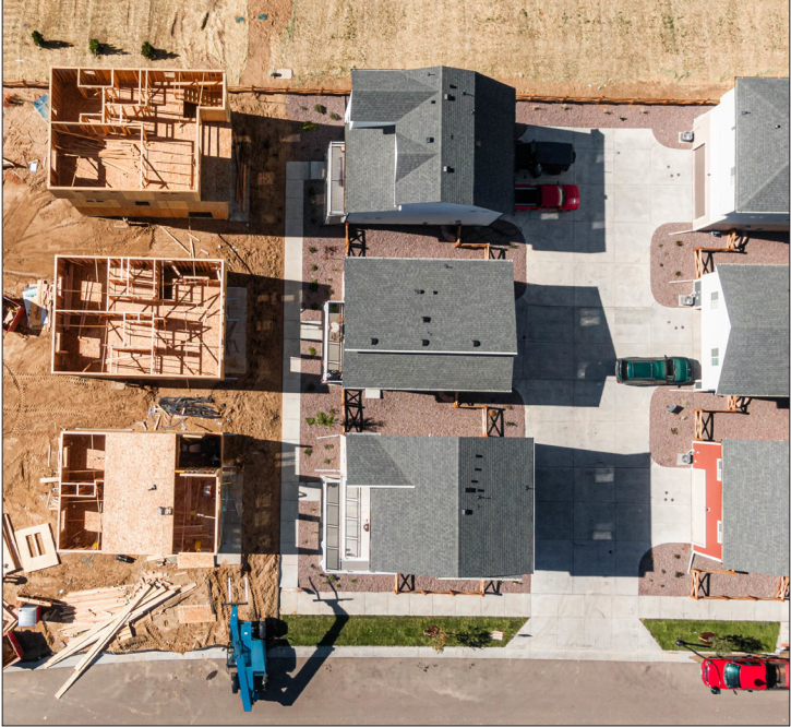
Newly constructed single-family homes in the Villages at Banning Lewis Ranch
