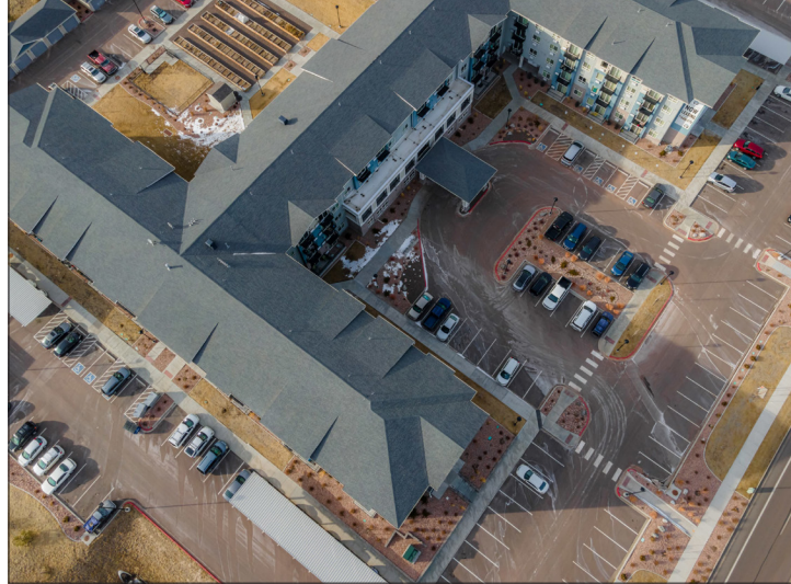
180-unit Traditions at Colorado Springs is an affordable senior community
